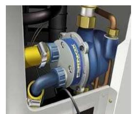
**5. Spajanje Powerflow Flushing Machine MKIII i Powerflushing Filtera na PPH Adapter (bojler)**
